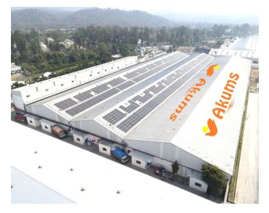
Contract development and manufacturing organisation (CDMO) Akums is making a large stride towards a greener and more sustainable tomorrow. Akums has successfully installed a 600 kWp on-grid rooftop solar power plant on its warehouse premises in Haridwar, Uttarakhand.
