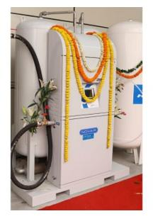
Uttam Group of Companies has installed 22 PSA plants for hospitals spread across Delhi. With a combined capacity of 13000 cubic metre per day, the oxygen generating plants aim to disrupt the way oxygen has been procured and delivered till now. The EN ISO: 13485 certified oxygen generation plants can generate on-demand oxygen by taking in atmospheric air and producing medical grade oxygen in quick and simple steps.
